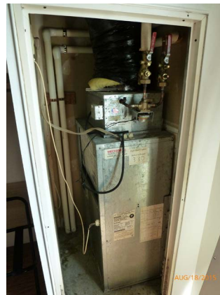
Photo of the previous unit installed versus the new upgraded VPAC unit in one of the Motel 6 guest rooms. Note the optional Hydronic heat coil installed on top and the air filter rack in front of the unit.
