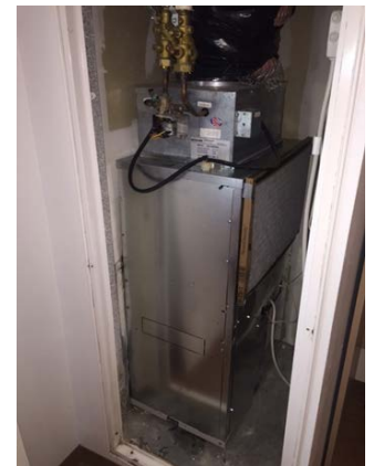
Photo of the previous unit installed versus the new upgraded VPAC unit in one of the Motel 6 guest rooms. Note the optional Hydronic heat coil installed on top and the air filter rack in front of the unit.
