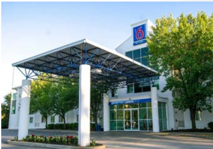
Exterior of the Motel 6 located in Colchester, Vermont.
