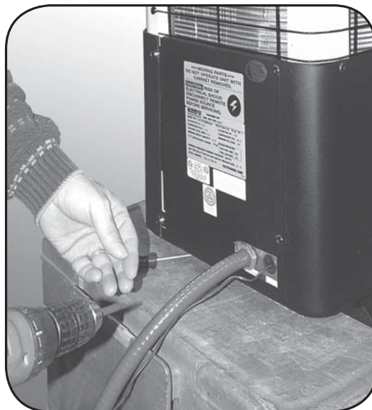
Figure 13 Fasten loose screws
