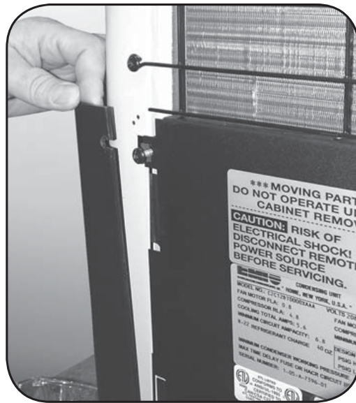
Figure 12 Replacing side panel
