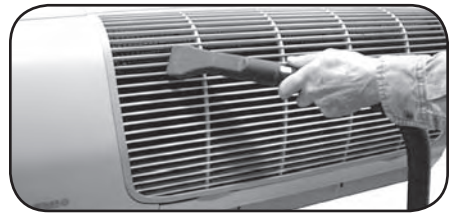
Figure 34 Clean front grille and coil with a vacuum
